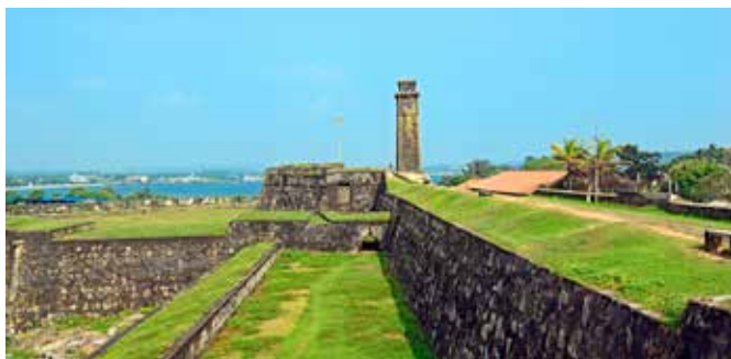
City clock tower, Galle
